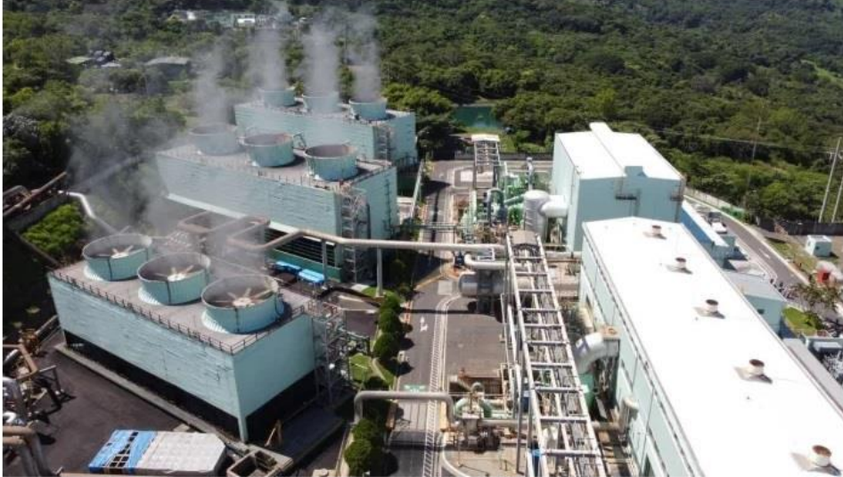
La Geo, the geothermal power station, where Bitcoin miners operate
